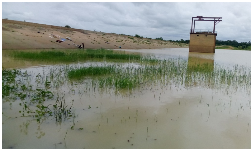
Figure 2: Sabke dam site at Yadi village, Mai'adua LGA on July 4 th 2021.
